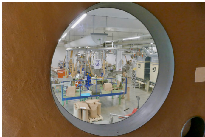
Figure 33: View of the filling station.
